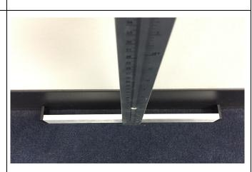
Use a level to ensure the height rod is vertically straight and plumb. While holding the level and height rod in place, insert a thin pencil or screw to mark the screw hole in center of the top hole. Next mark the screw holes for the center and bottom holes.
